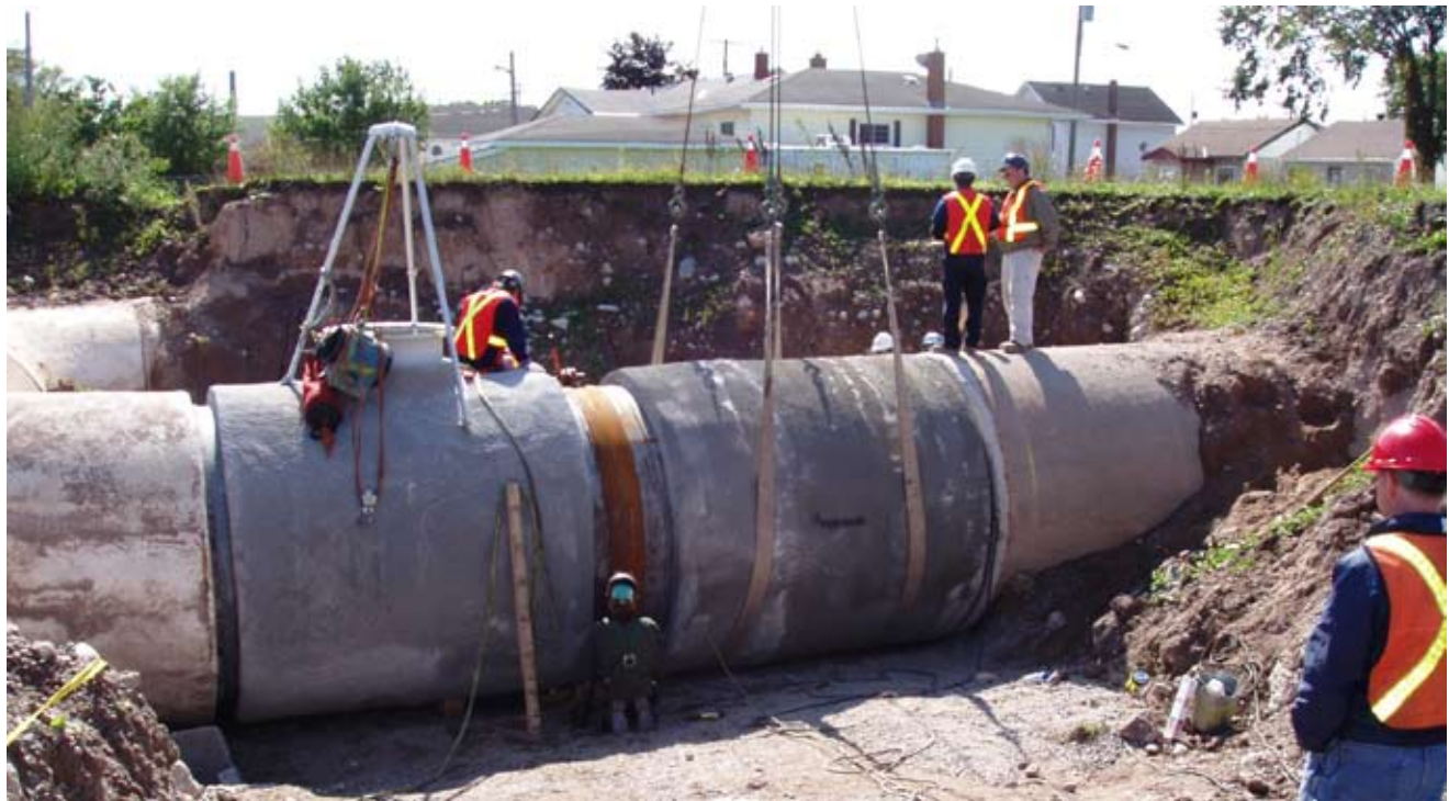
Retention Main at Steelton Pumping Station on 2nd Line West
